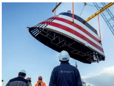
Precision work down to the centimeter when installing the funnel
