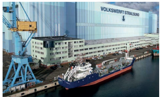
Fabrication hall 290 at Volkswerft Stralsund
